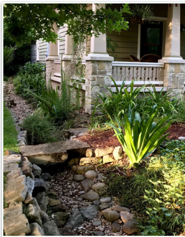
A bioswale in an old Houston neighborhood. Photo courtesy of the Houston Chronicle
